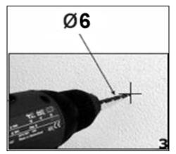
**3)** Using a drill bit with a 6 mm diameter, make holes in the wall on the positions that you have marked in step 2.
